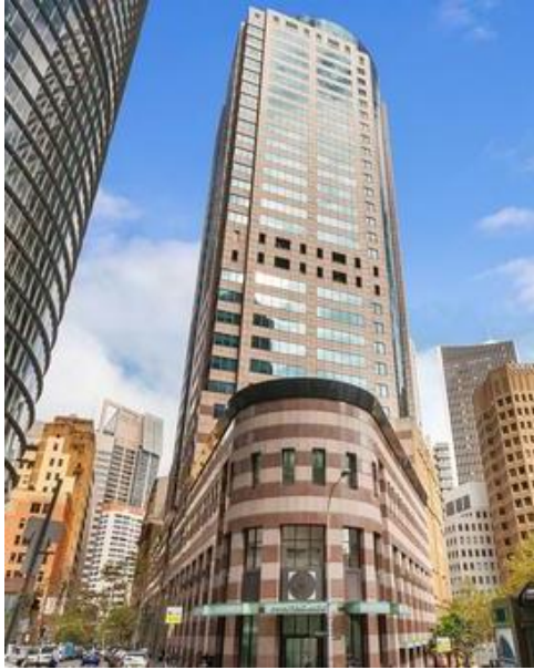
The Wintergarden, 1-15 O'Connell Street
