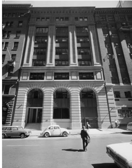
September 1971. The arch at right has been altered to provide driveway access to the new basement carparking. Source: SLNSW: Max Dupain, Call no. ON 558/Box 82/nos. 580-594, contact sheet image 36537_09
